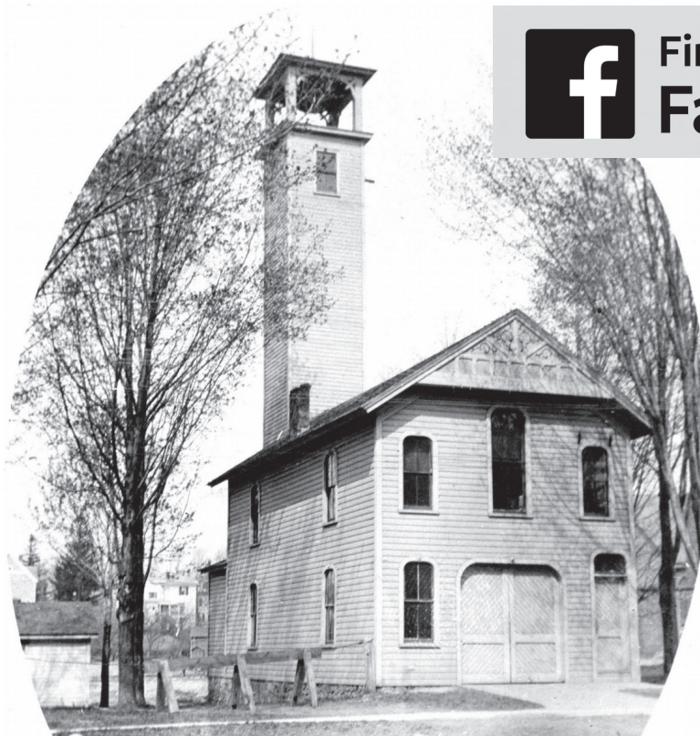
This is Wolcott’s old fire hall that was once on New Hartford St. In 1912 it was moved to Leavenworth Ave and converted into a residence. It has been in the Trine family since 1960 and is now owned by Craig Trine.
